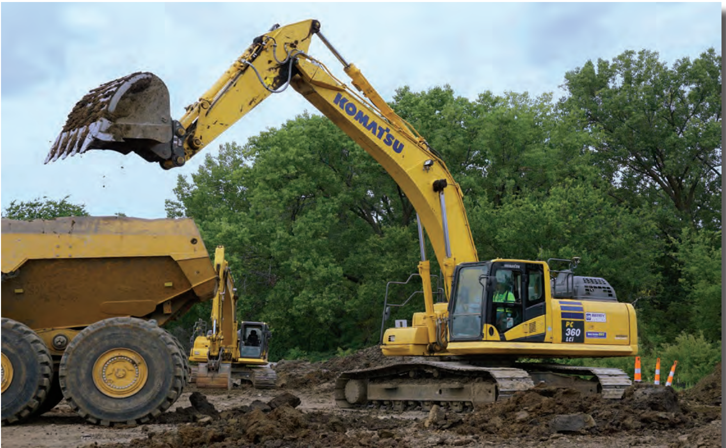
Two PC360's doing infrastructure work on a mixed use commercial development in southwest Topeka. The machine in the foreground is an "i" model designating the built-in-3-D GPS connectivity.
