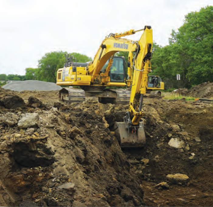
A PC360LCi doing infrastructure work on a mixed use commercial development in southwest Topeka.
