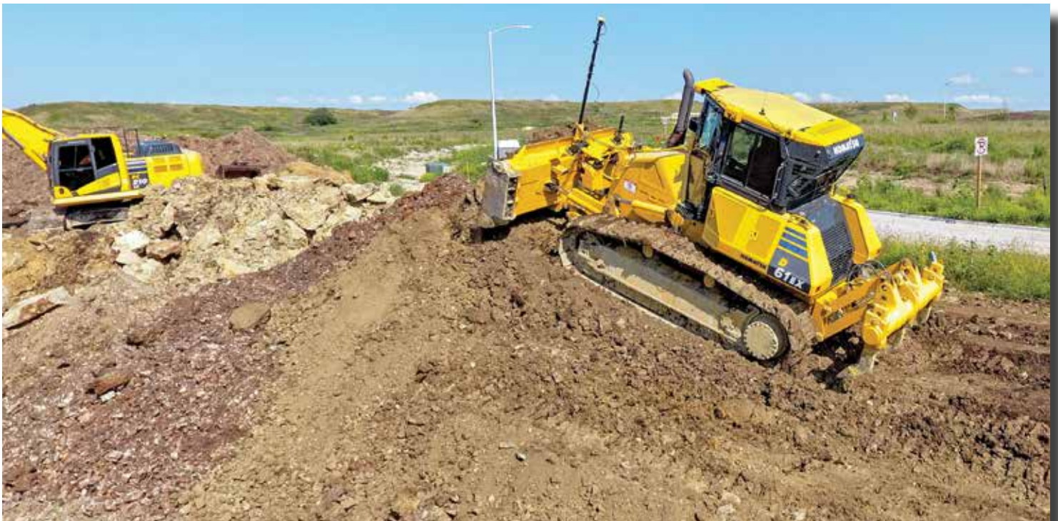
Using a Komatsu D61PX dozer equipped with an aftermarket GPS system, a Gideon Excavating operator grades a building pad.
